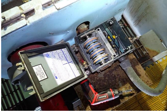
Photo 04: Interior of Housing Showing No Corrosion on Rotary Cam (Personal Photo)
